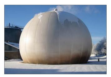
Figure 3: The gas buffer storage of 1000 m<sup>3</sup>
